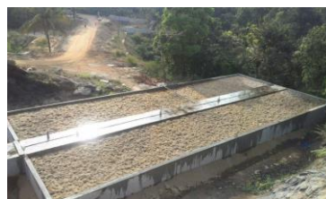
20,000 m 3 /h capacity Biofilter
