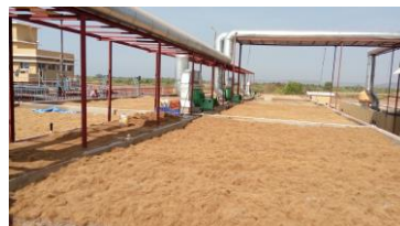
64,000 m 3 /h capacity Biofilter
