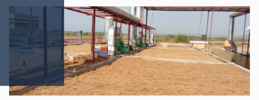
The EES-BioGuard Biofilter is a traditional, fixed-bed system that uses a single-storey biofilter to treat odorous air.
