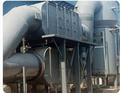
The EES-Rapid High-Rate Biofilters are engineered to handle high volumes of odorous emissions within a compact system.
